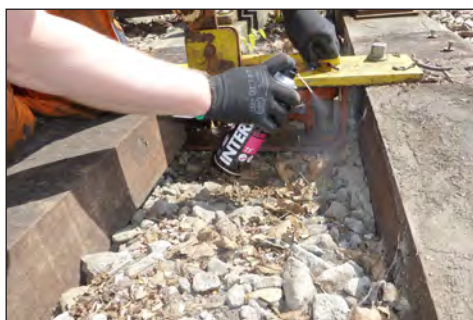
Lube TF sprayed into pull arm pivot
