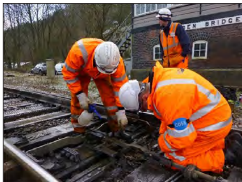
Clean all moving parts with Degreaser EM30+ & Metal Clean
