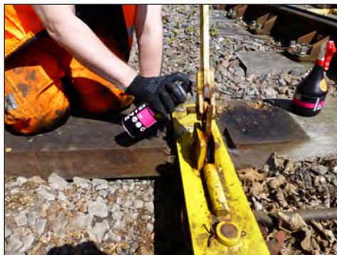
Lube TF sprayed into pull arm pivot
