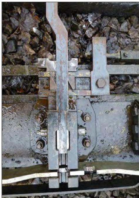
Lube TF sprayed into pull arm pivot
