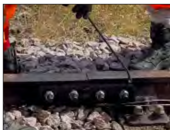
Lube EP into fishplate with Backpack
