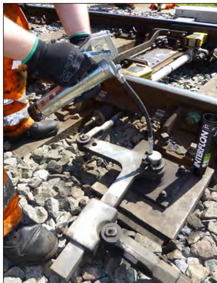
Application of Grease MP1 into crank boss & pins
