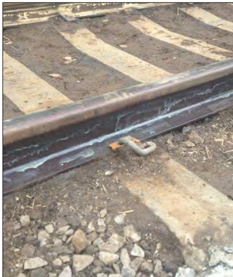
Grease OG sprayed onto rail web
