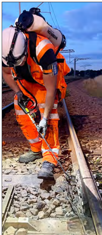
Lube EP into fishplate with Backpack
