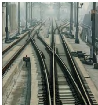
Typical switch layout in Shanghai
